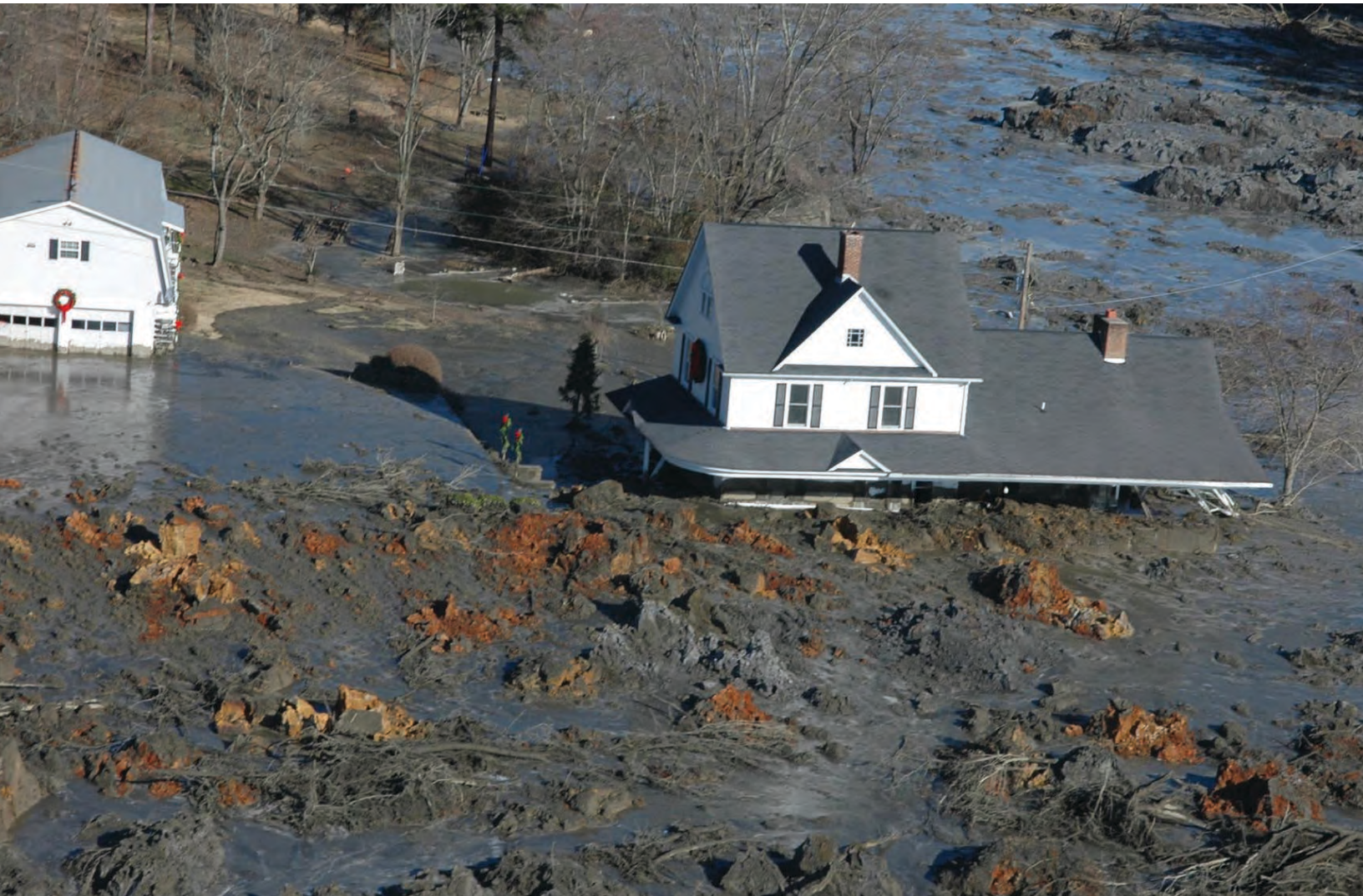
Coal ash spilled from the TVA Kingston Power Plant covered 300 acres and damaged 40 nearby homes.
