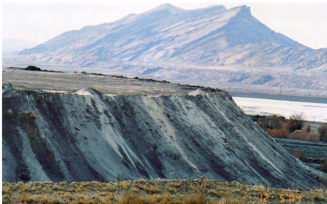
Coal ash ponds from APS' Four Corner's Power Plant rise more than 100 feet above the arid Navajo Reservation.
