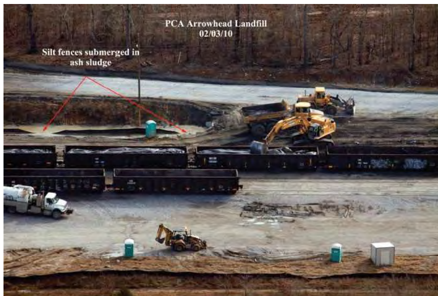
Figure 6: Fly ash unloading from rail cars at Arrowhead Landfill, AL Photo courtesy of John Wathen, Hurricane Creekkeeper, Waterkeeper Alliance
