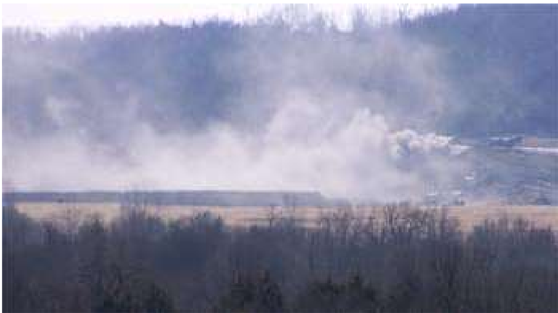
Figure 3: Fly ash dumping at CCW landfill in Bokoshe, OK
