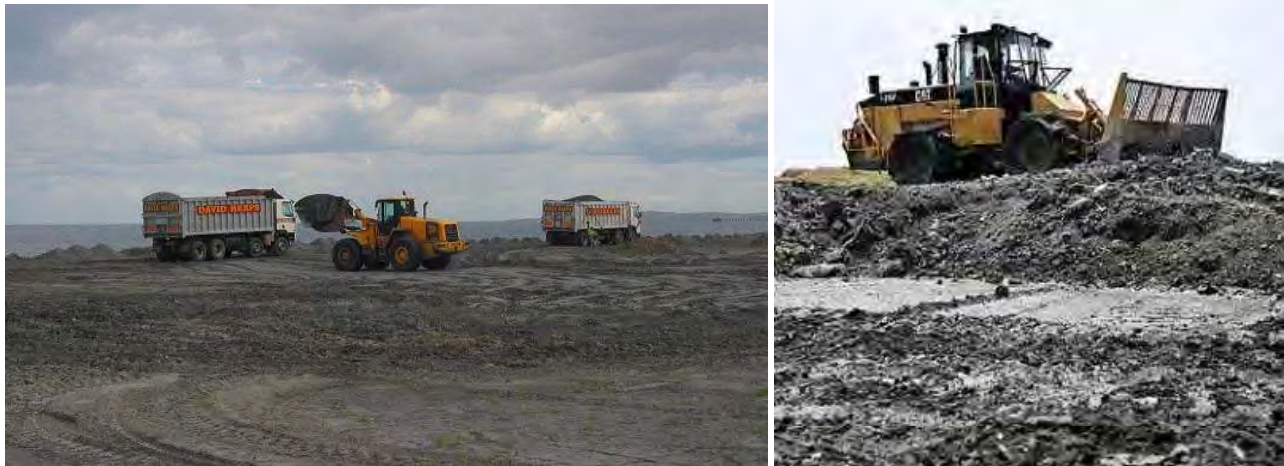
Figure 7: Heavy-duty equipment at fly ash landfills
